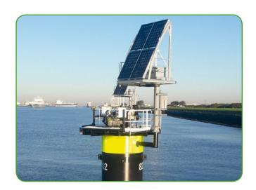
Straatman was the first company in the world that supplied quick release mooring hook units with integrated capstans powered by solar panels, to be used on mooring dolphins.
